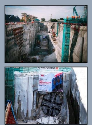
PROJECT PROJECT MASS RAPID TRANSIT LALUAN 2 SUNGAI BULUH-SERDANG PUTRAJAYA (SSP) THE CONSTRUCTION AND COMPLETION OF EXCAVATION WORKS, ROCK STRENGTHENING STEEL STRUTTING AND OTHER ASSOCIATED WORKS FOR STATION BOX, ENTERANCE AND PAID LINK AT CHAN SOW LIN
