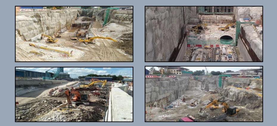
PROJECT PROJECT MASS RAPID TRANSIT LALUAN 2 SUNGAI BULUH-SERDANG PUTRAJAYA (SSP) THE CONSTRUCTION AND COMPLETION OF EXCAVATION WORKS, ROCK STRENGTHENING STEEL STRUTTING AND OTHER ASSOCIATED WORKS FOR STATION BOX, ENTERANCE AND PAID LINK AT CHAN SOW LIN
