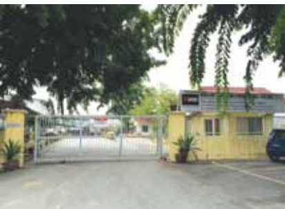
Production facility located at Ulu Yam, Selangor
