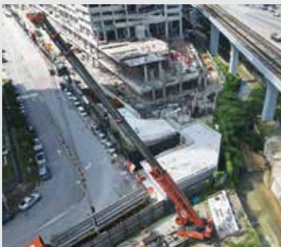
Road upgrading works along the Cheras-Kajang Expressway
