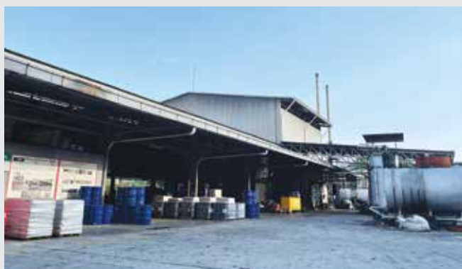
Production facility located in Ulu Yam, Selangor
