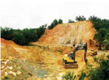
Drill and blast operations at a gold mine in Pahang
