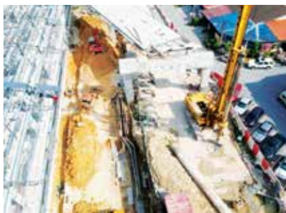
Construction of an elevated road at Cheras, Kuala Lumpur
