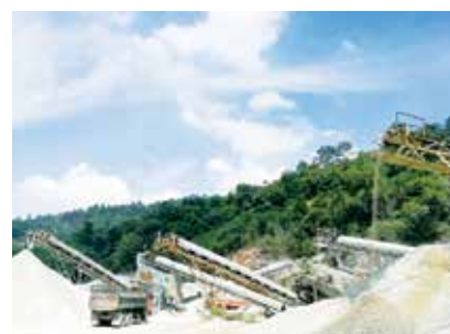
Quarry operation at Nilai, Negeri Sembilan
