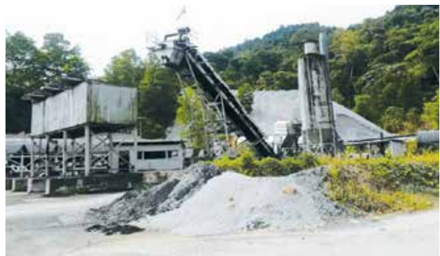
100 metric ton per hour capacity drum mix plant at Bidor, Perak
